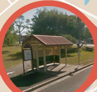
ANZAC PARK BUS STOP ON CHEAPSIDE STREET, MARBOOROUGH
